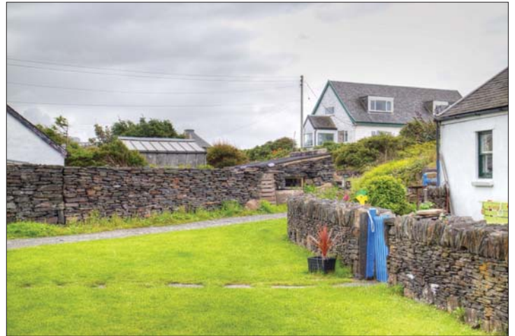
Dry-stone slate boundary walls
