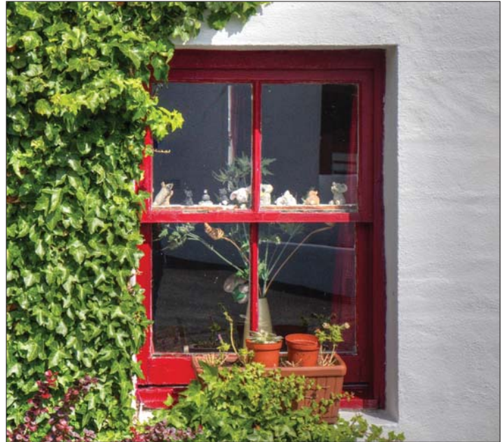
Traditional sash and case window with slim astragals—an asset to the conservation area
