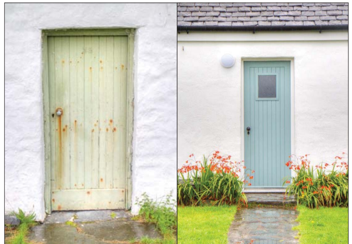
Traditional and new doors showing different proportions
