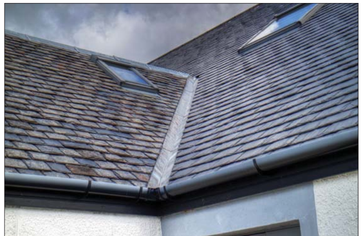
New and reclaimed slates on Community Centre
